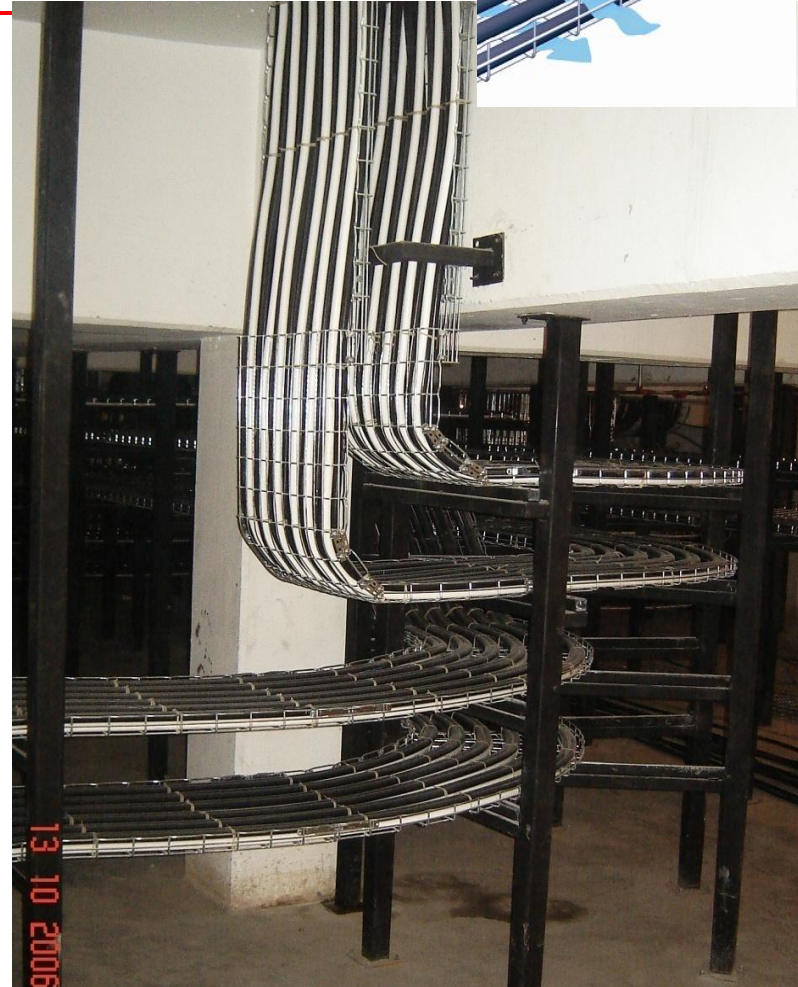
Has the same solidity but is more flexible than standard cable tray
